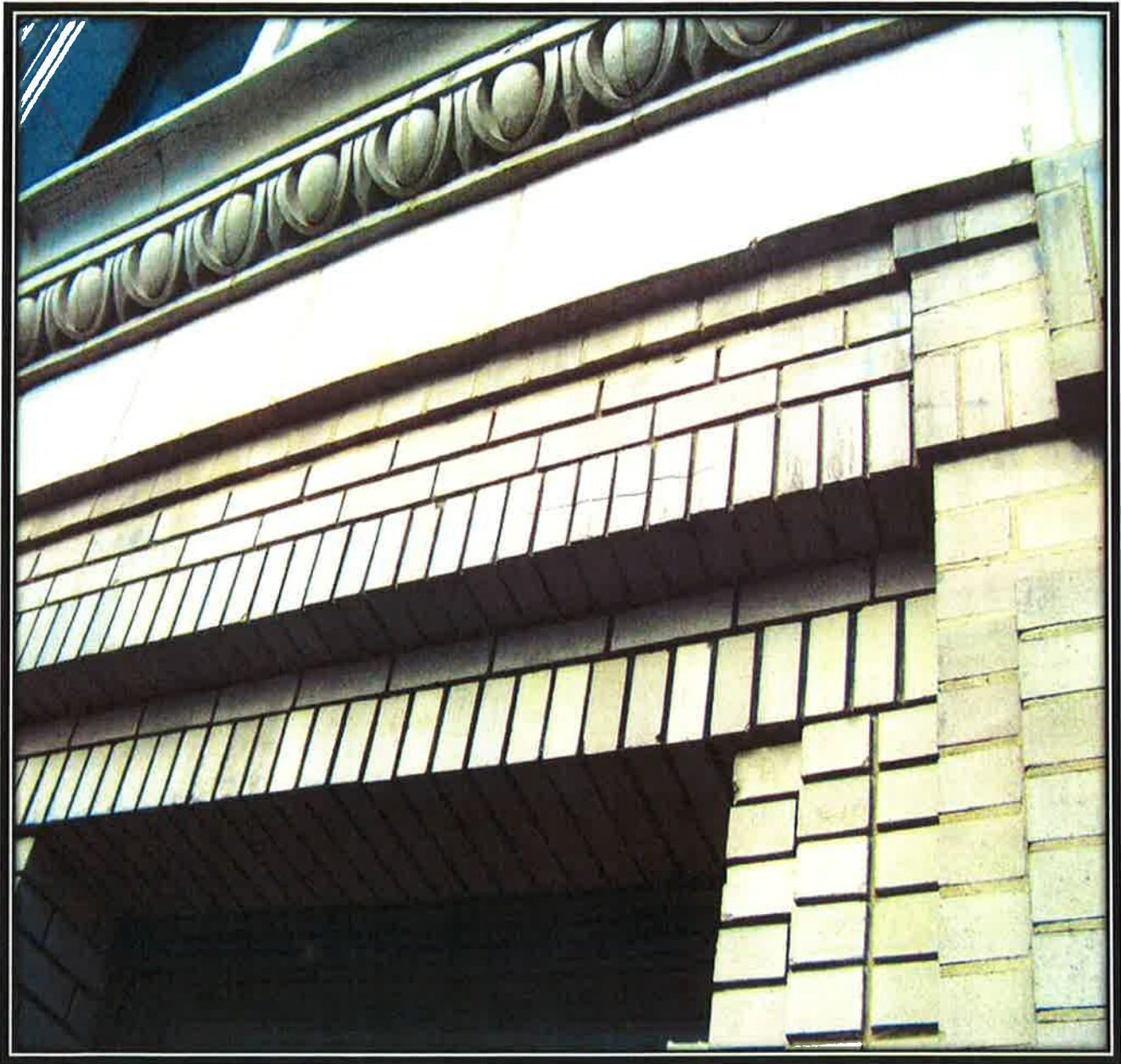
Example of brick lintel to replace
