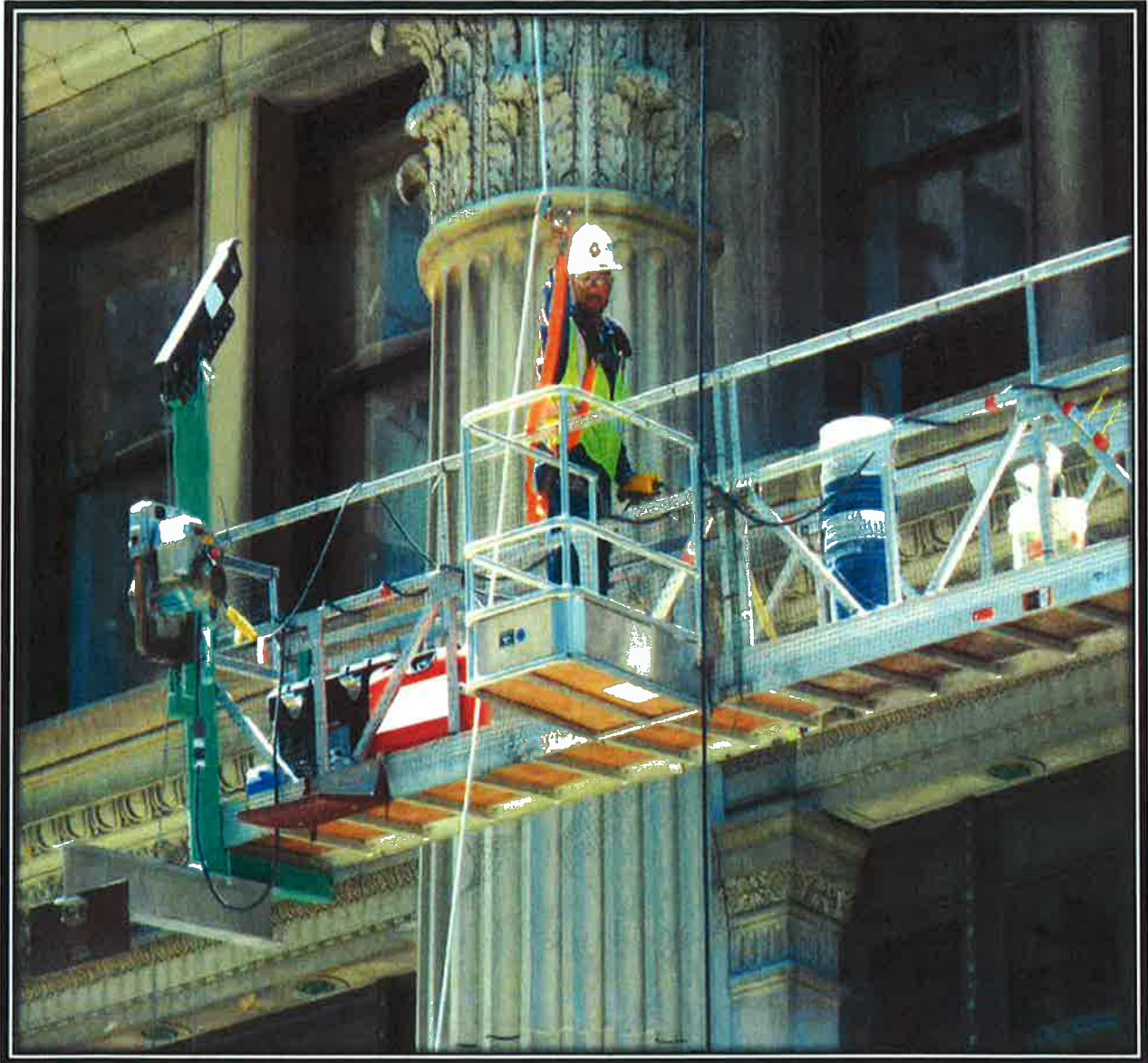
Porch bracket example depicting extending upper level work access
