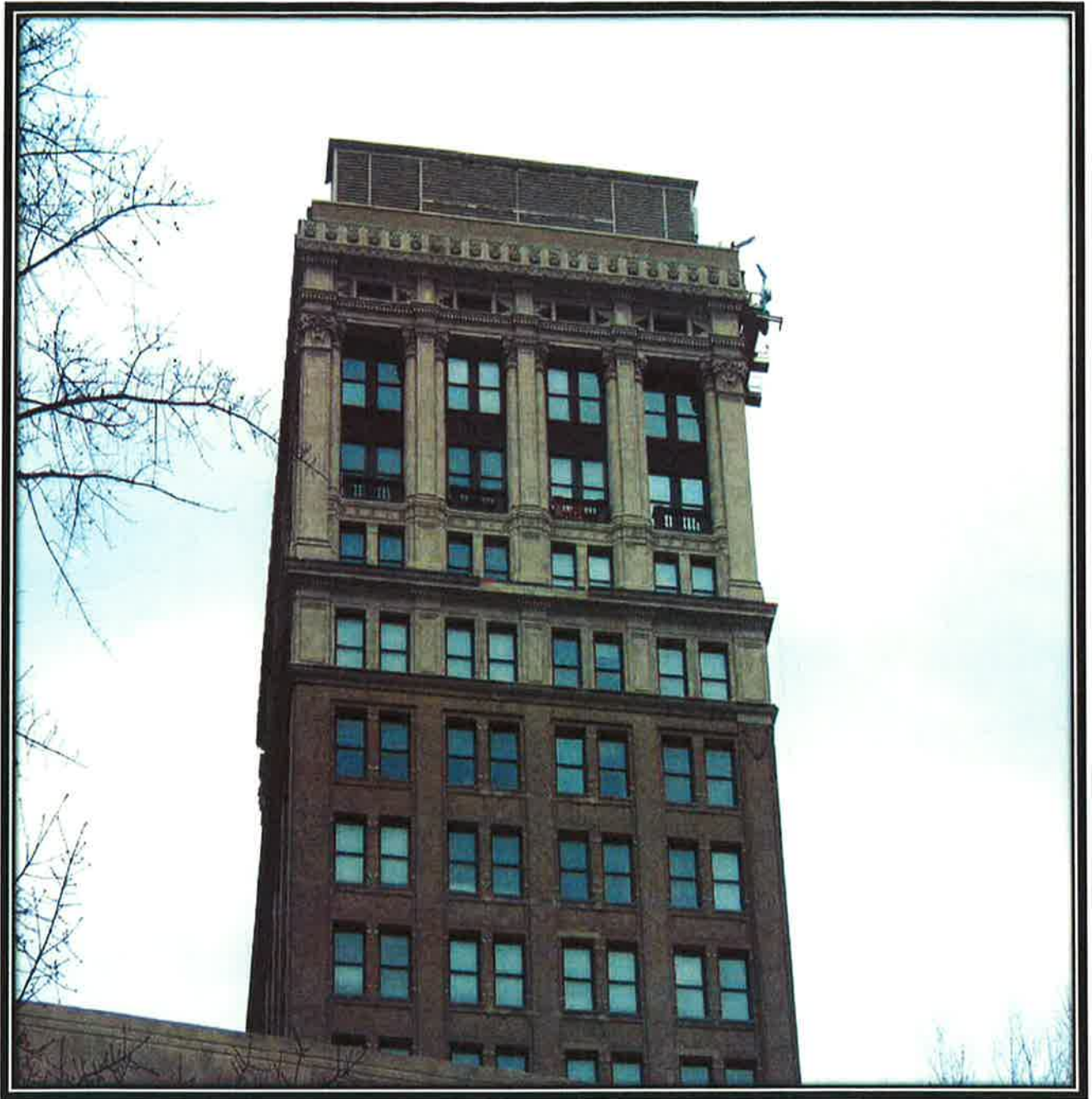
Completed project picture except brick hoist drop
