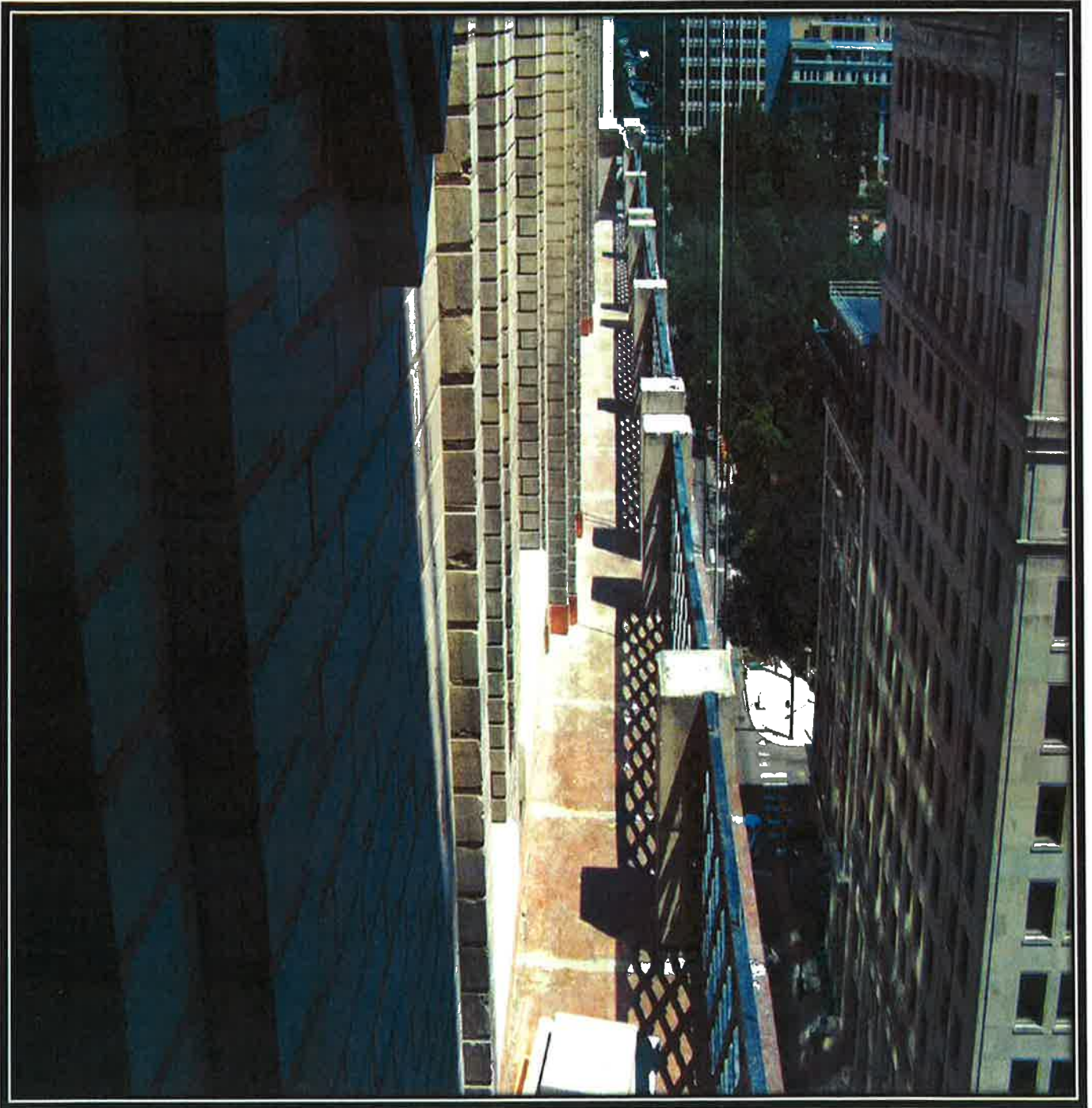
Upper level balcony reconstruction
