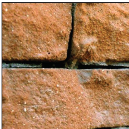
Sandblasted – this close-up of masonry subjected to an ill-conceived abrasive cleaning process shows damaged mortar joints and exposure to weather of the soft inner body of the brick.
