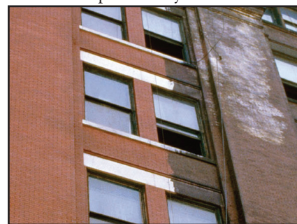
Acidic cleaners – A restoration cleaner containing a small amount of hydrofluoric acid removes decades of atmospheric staining from the clay brick and terra cotta masonry of the County Records Building, New York City.
