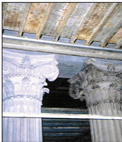
Poultice Cleaning – This limestone column cap (L) in the Tennessee State Capitol, soiled by decades of tobacco smoke and dust was cleaned with a poultice stain remover. A similar cap (R) waits for the same treatment.
