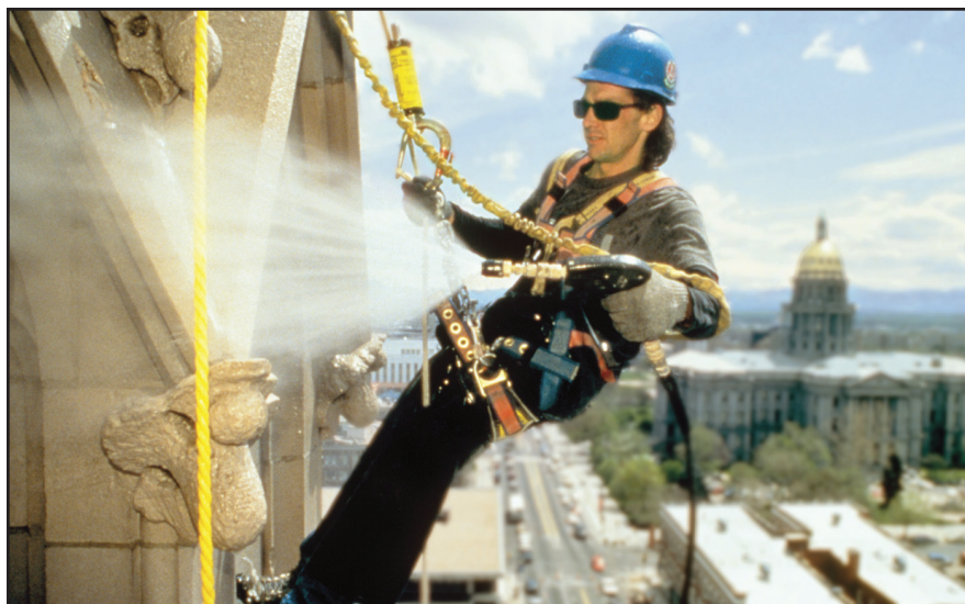
Pressure Washing – A technician uses a pressure washer to flush spent chemical cleaner and dissolved soiling from the limestone masonry of Denver's Cathedral of the Immaculate Conception. Pre-wetting is an important first step in the cleaning building with a combination of pressure-washing and chemicals.
