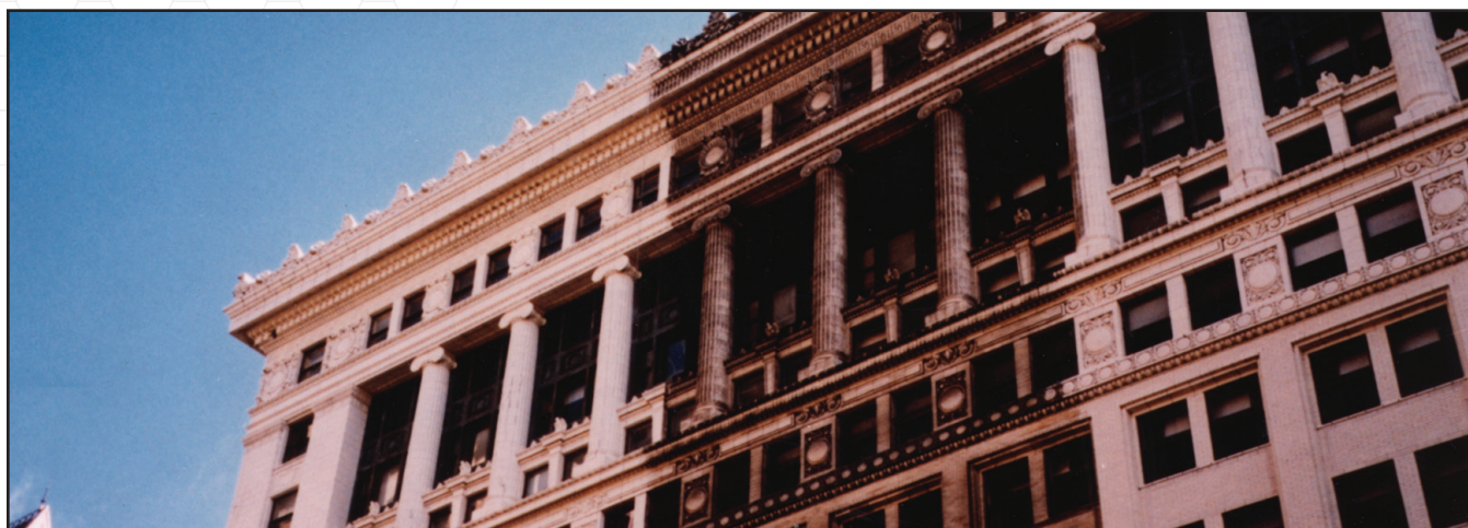
Acidic cleaner – The limestone masonry of the Insurance Exchange, Chicago, was cleaned with an alkaline restoration cleaner. The cleaning contractor temporarily left the 30-foot wide strip of uncleaned masonry to show the difference a good cleaning makes.
