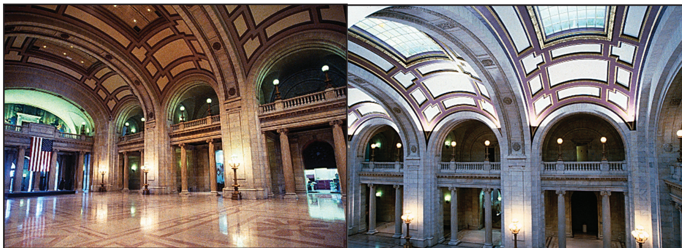
Neutral cleaning before & Neutral cleaning after – Decades of tobacco smoke stained the sugar-white Colorado marble of the Cuyahoga County Courthouse's ceiling and walls. Workers used a neutral-pH restoration cleaner to restore the interior's original appearance.
