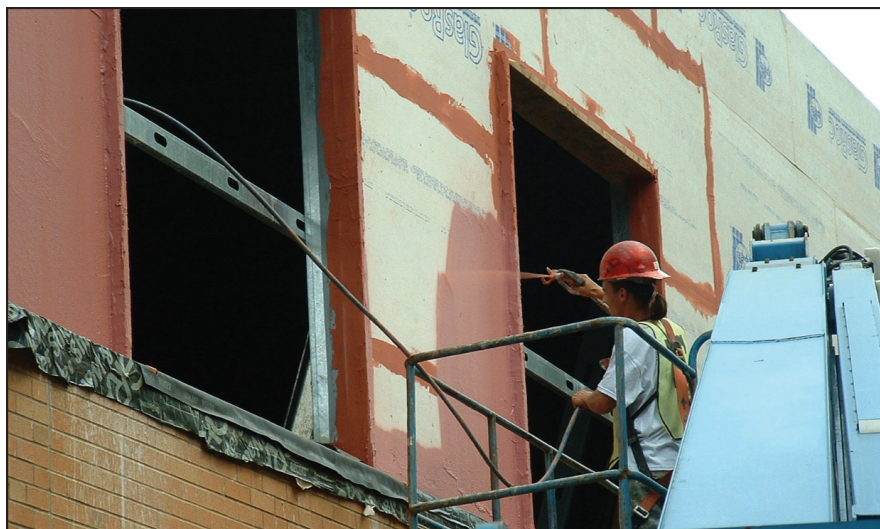
Application of a spray-applied liquid air barrier over a gypsum-based sheathing, note the use of self-adhering sheet membranes used as flashings at the shelf angle.
