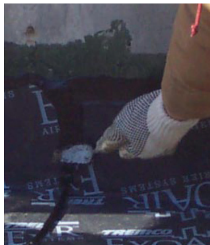
Detailing of laps in the flashing of an air barrier.
