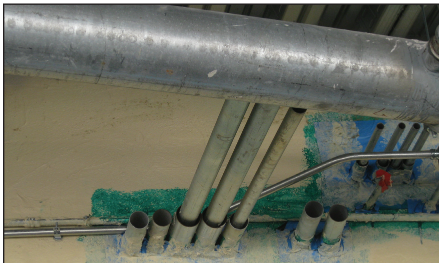
Achieving “continuity” of the water-resistive barrier can be difficult and detailing must be considered at locations such as pipe penetrations.
