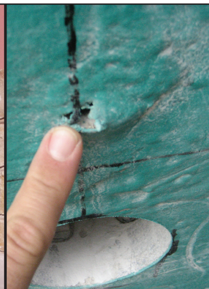
Small defects in air barriers can lead to leaks, energy loss, and other problems.
