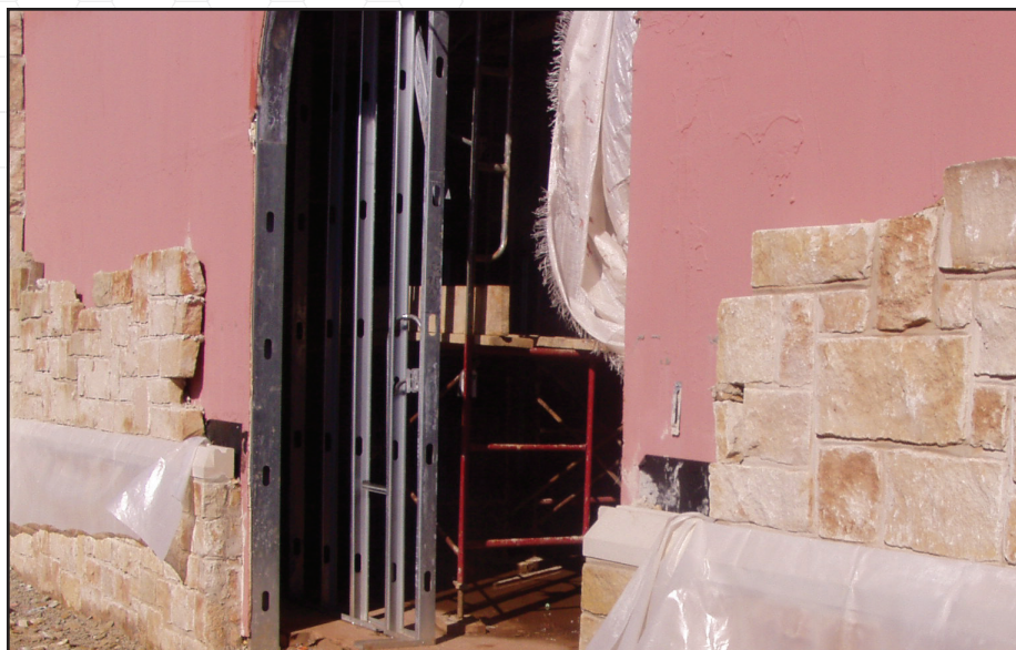
Air barrier installed as a drainage plane in a cavity wall system.
