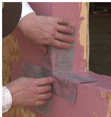
Reinforcing a corner detail for a liquid applied air barrier which will also act as a flashing.
