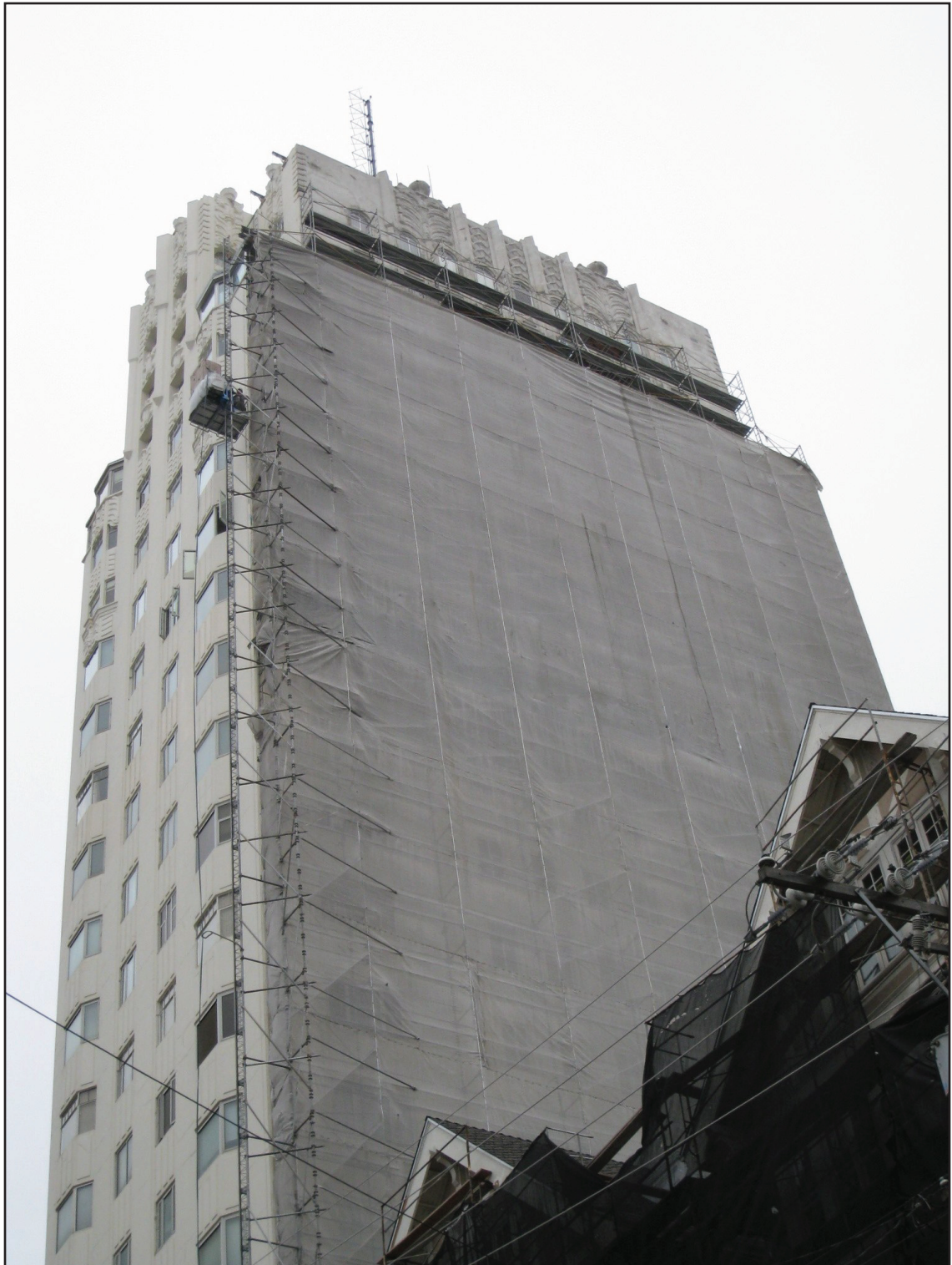
20 story scaffolding erected on the west wall, fully enclosed.
