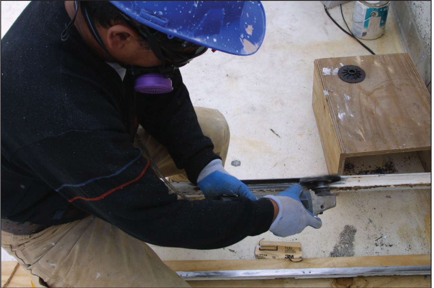
Window refurbishment was tedious and labor intensive. Example of the work required to restore the windows.
