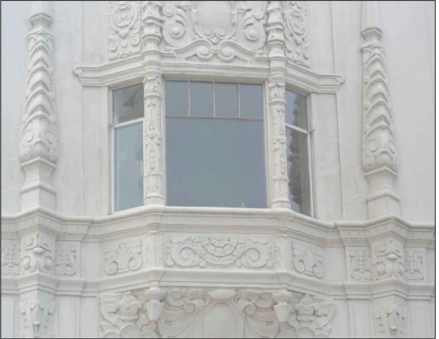
Completed area. Note the intricate detailing and ornamentation. The four vertical elements of the window are made of GFRC.
