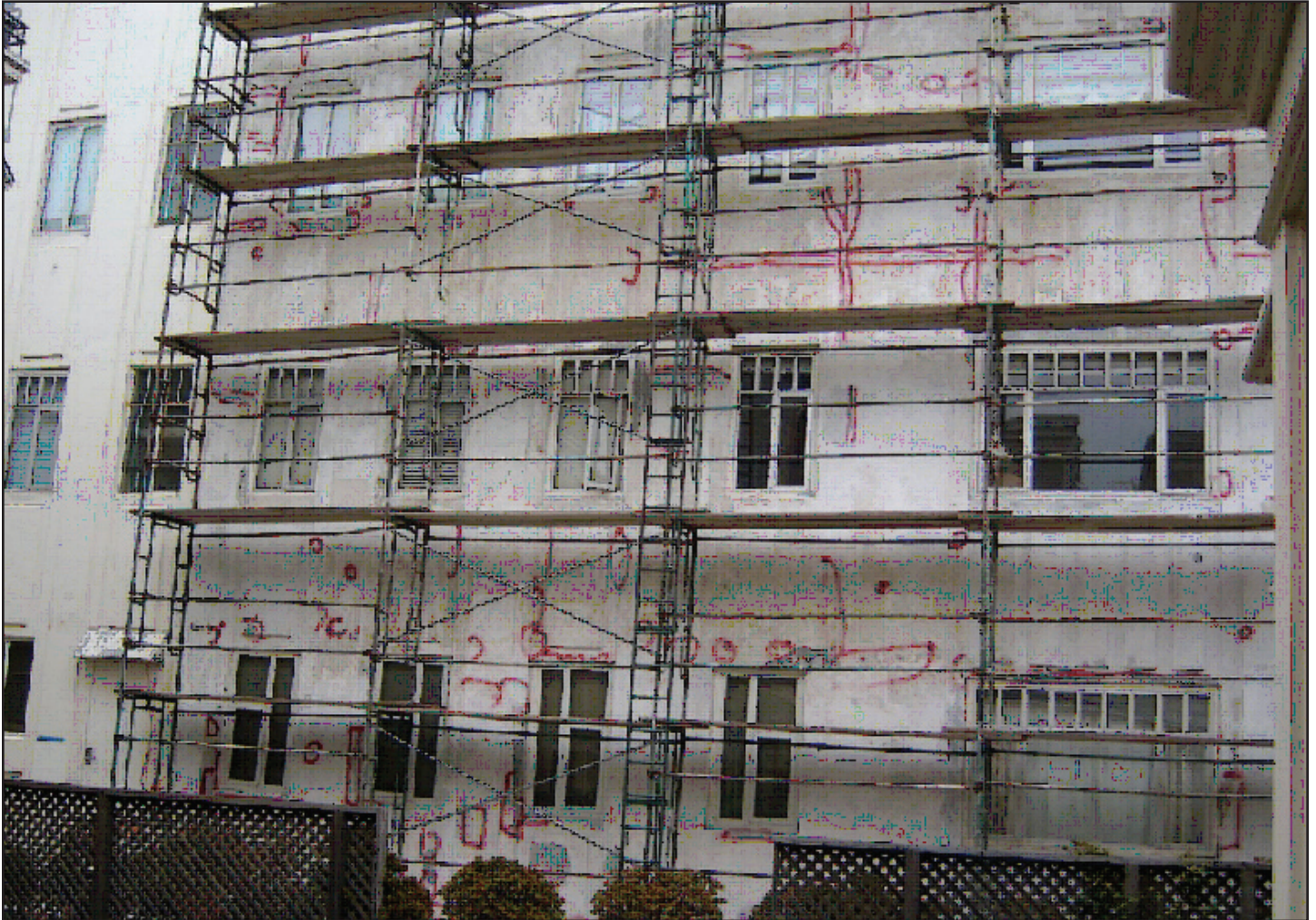
Mock-up phase, coating removed and delamination and cracks identified.
