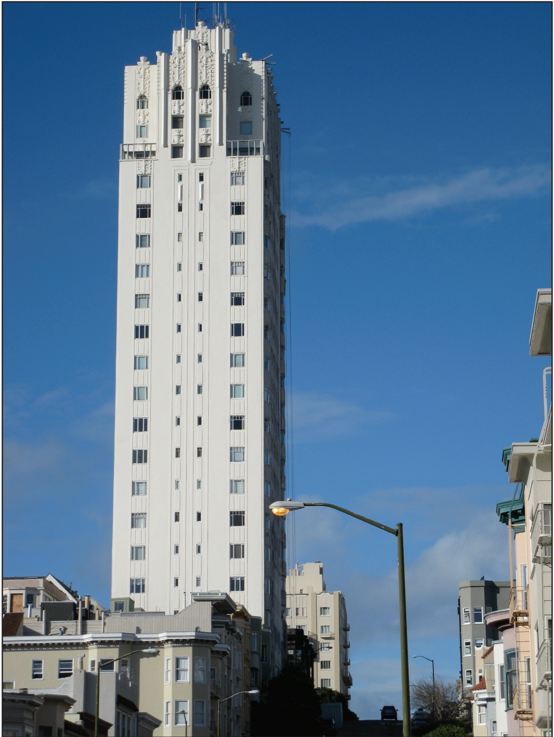
South elevation, looking North.
