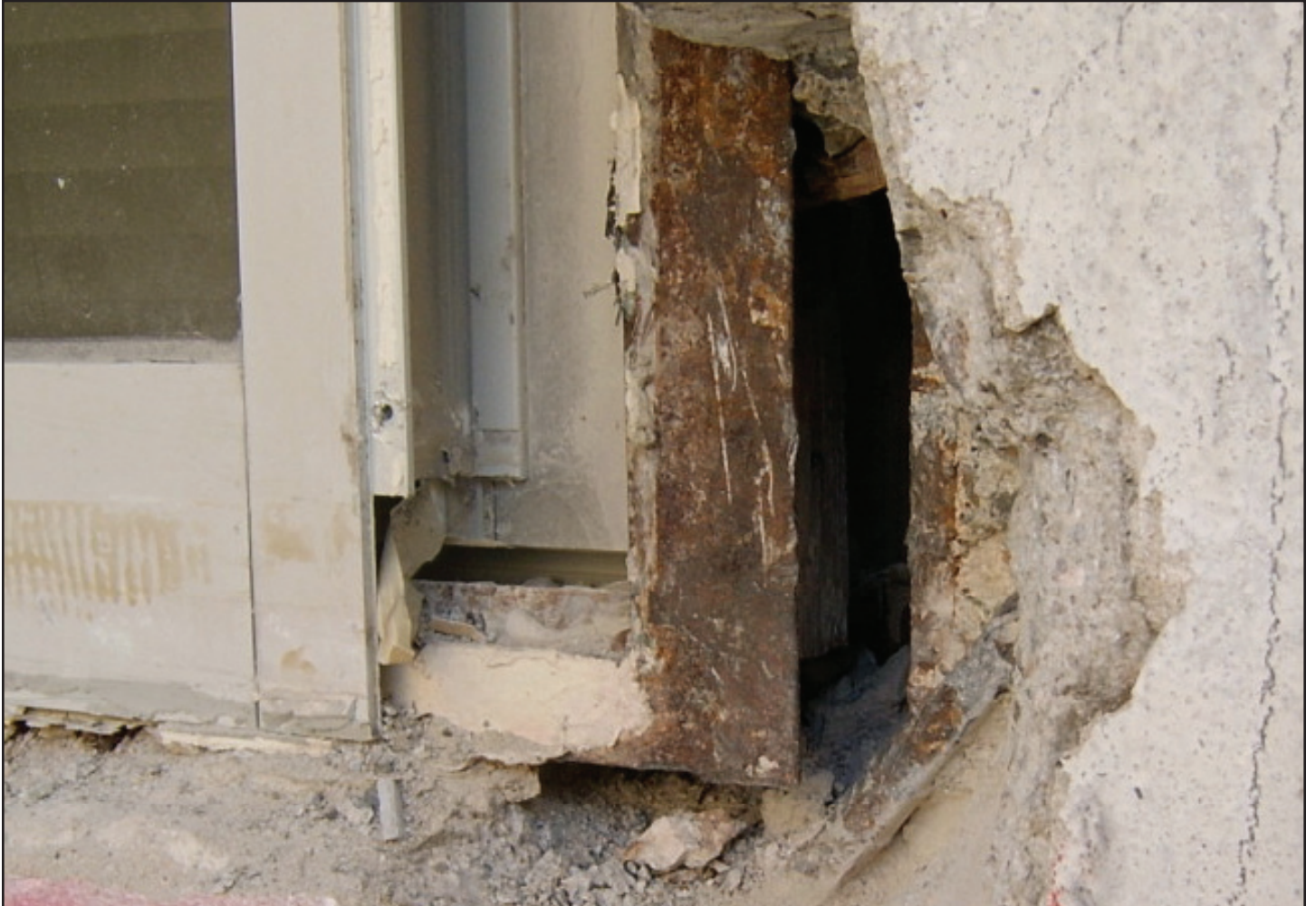
Good example of spalling caused by the window steel flange corrosion.
