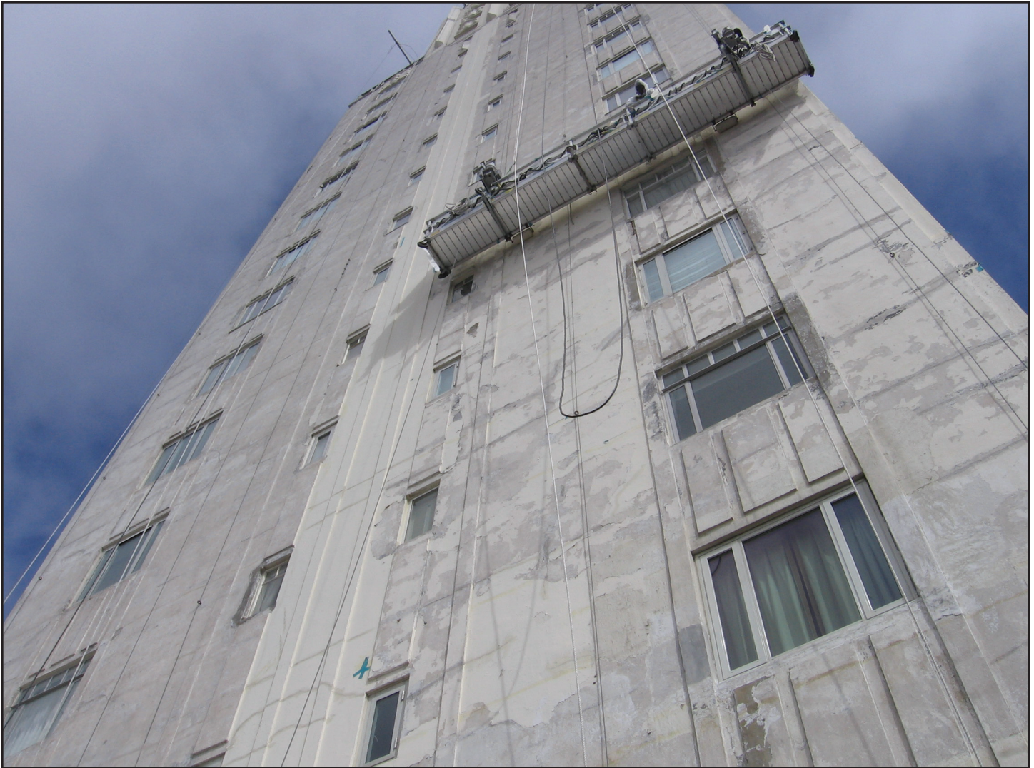
Coating removal required several passes using different methods to complete.
