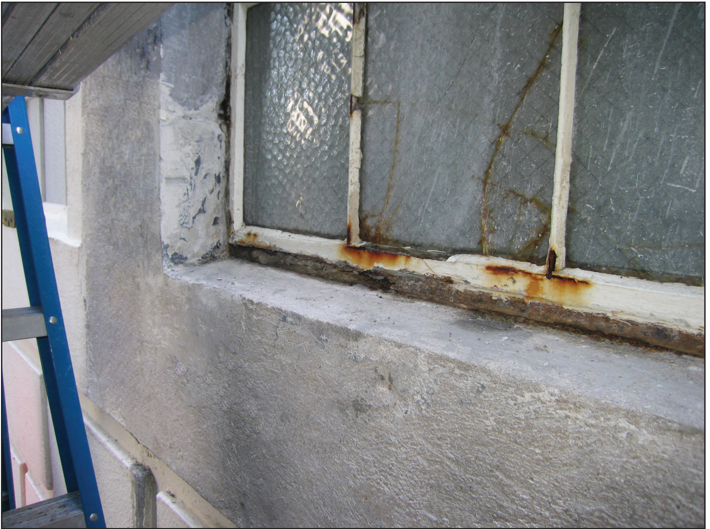
An old window showing signs of its age.
